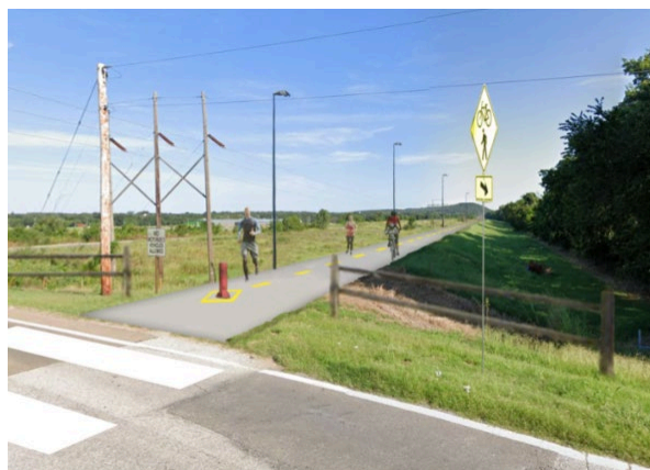
Figure 20. Concrete Trail on top of Levee on the West Bank
