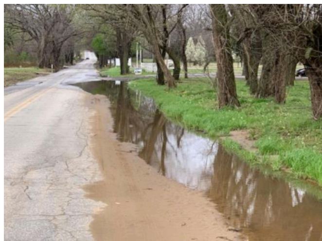
Image 5. Standing Stormwater along W. 81st Street currently used by cyclists, roadway pavement condition index 42
